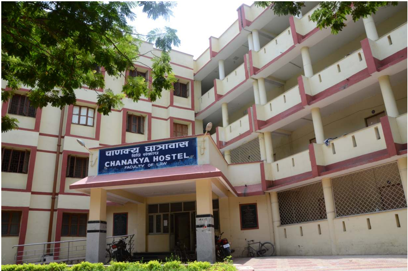
Newly constructed Chanakya and Ramanujan Hostels
