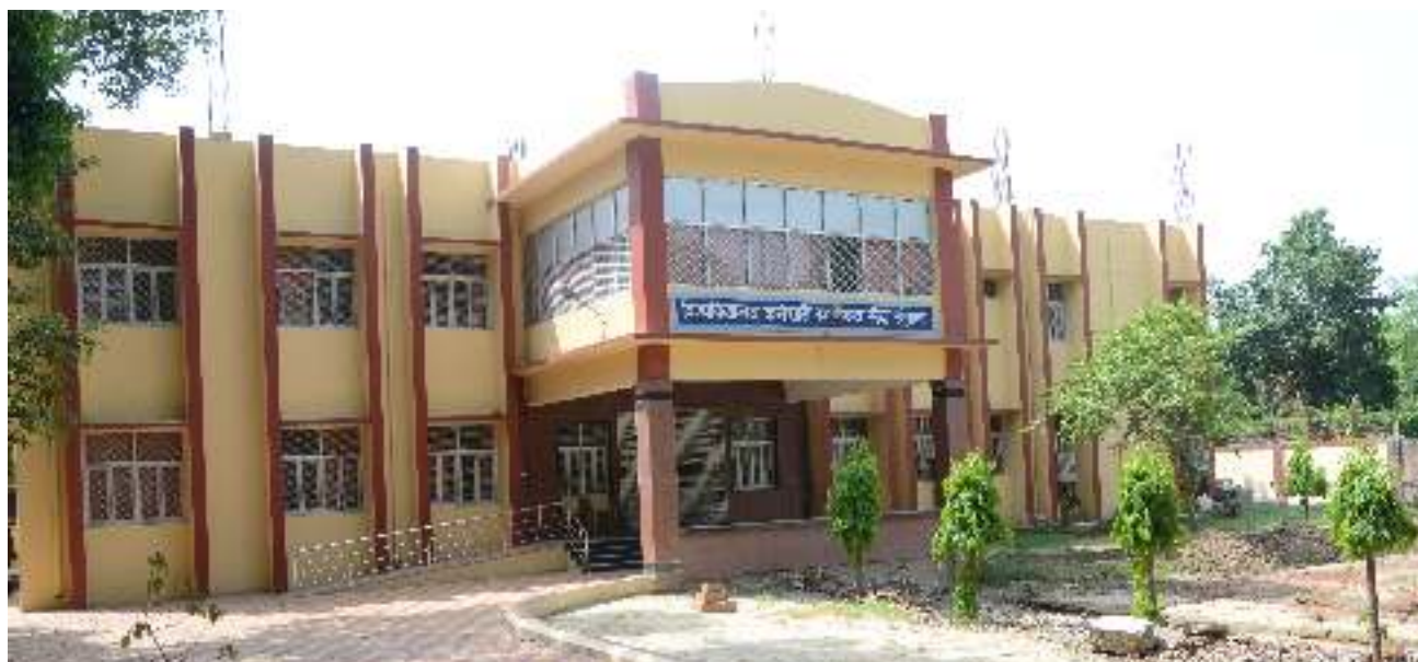
Newly constructed building University Employee Health Care Complex
