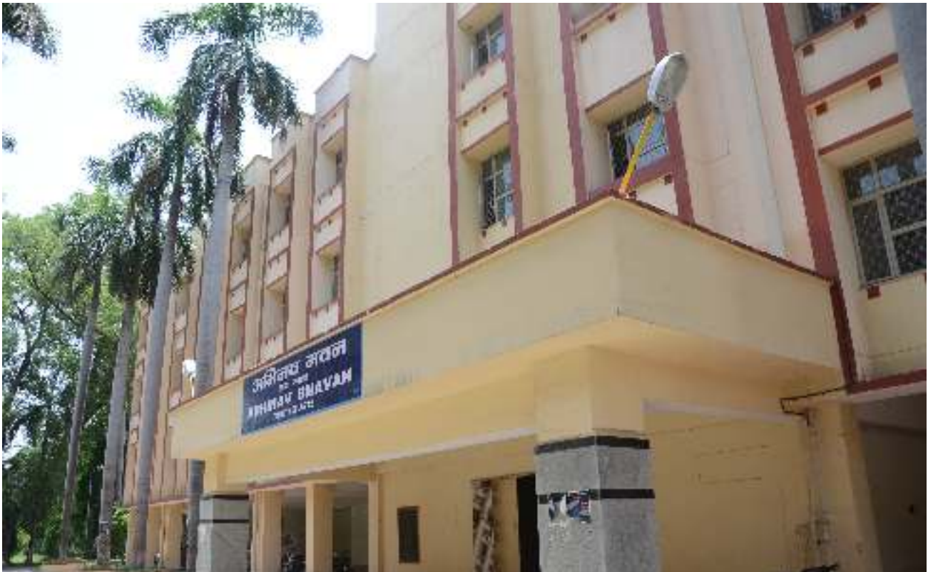
Newly constructed Academic Block-"Abhinav Bhawan" of the Faculty of Arts
