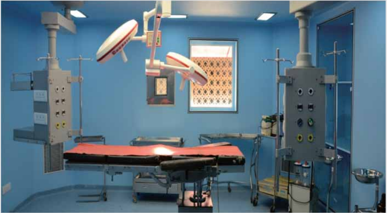
Modular Operation Theatre, Sir Sunderlal Hospital, BHU
