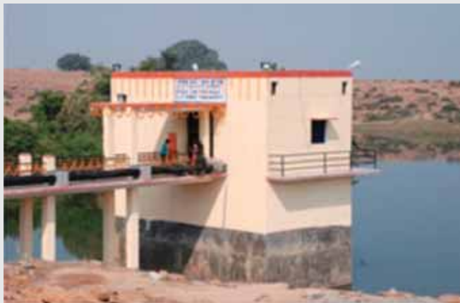
Intake Well and Pump House
