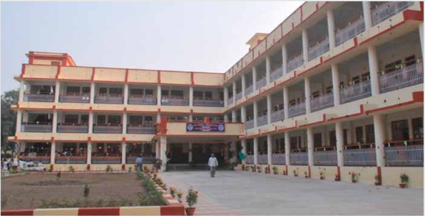
Kendriya Vidyalaya Main School Building
