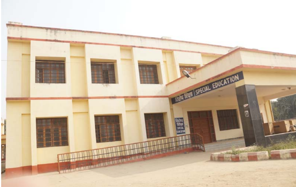
Photo 6: Faculty of Education New Building at Kamachha (Above it one more floor is under construction with the funds of School of Education of the Faculty at present )
