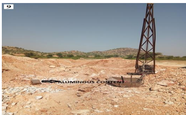
Fig 9. Quarry of high alumina-rich clay deposit (Gangrar region, Rajasthan.)
