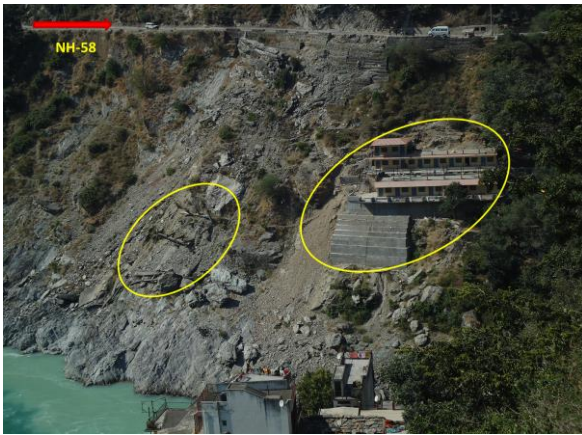
Fig.8. House present in danger condition in middle right part of the photograph and foundation of another house damaged in middle left of the photograph due to L_1 landslide.
