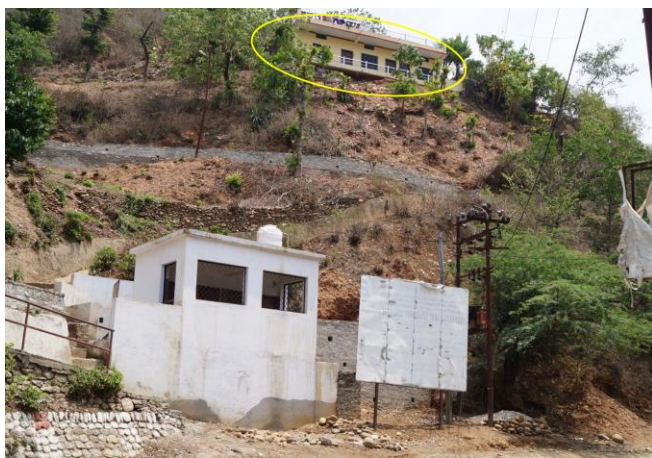
Fig. 12. In this photograph material below the house has moved down due to L 4 landslide and house is in danger condition. House is marked by ellipse.
