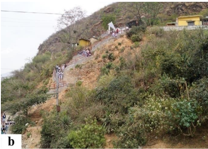
Fig.11 b. At places plantation of Rambans (cactus) has been done for landslide treatment.
